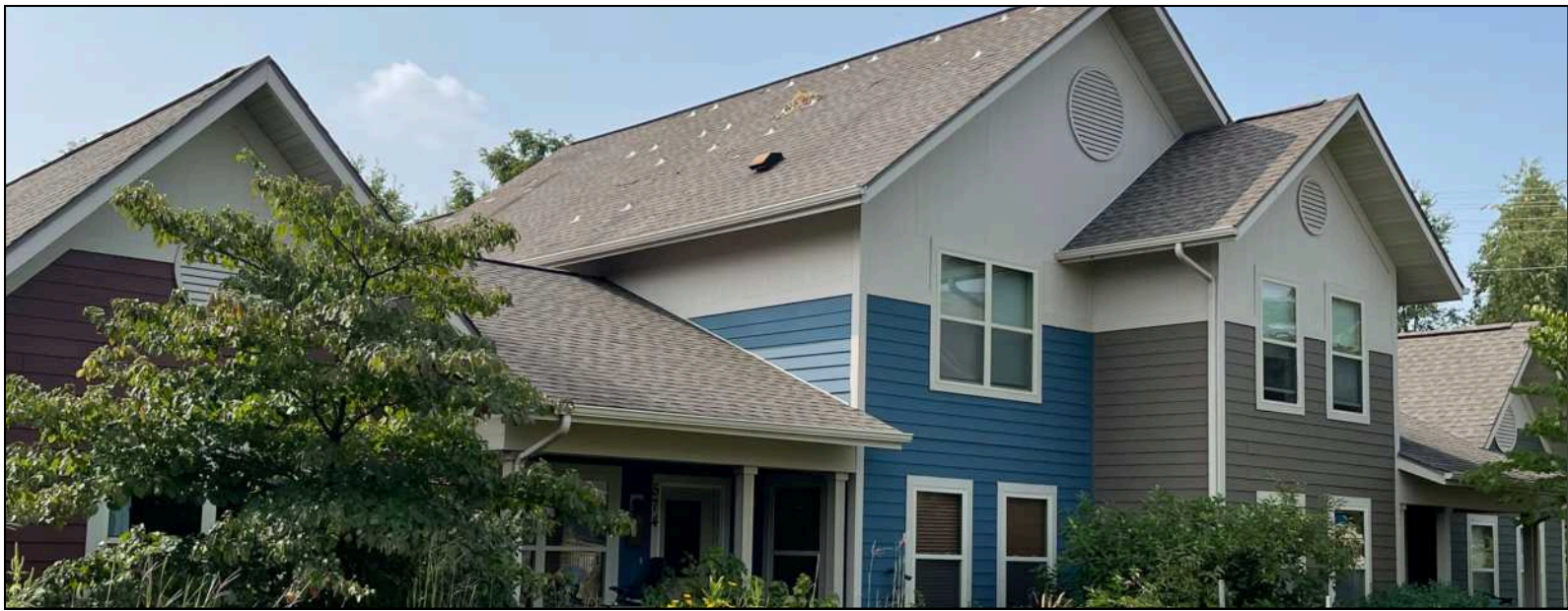
Pictured: Troy Gardens roofing project.
